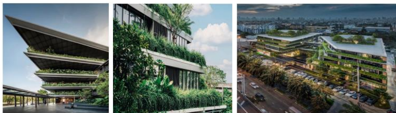
Figure 4: Proposed new acquisition – The 111 Praditmanutham office building
